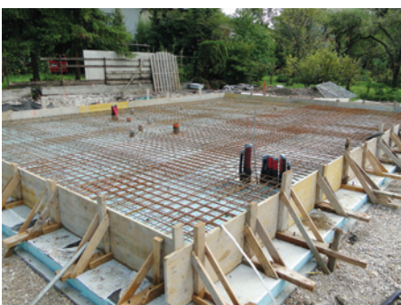
14: Armatura na blazini XPS Seismic
