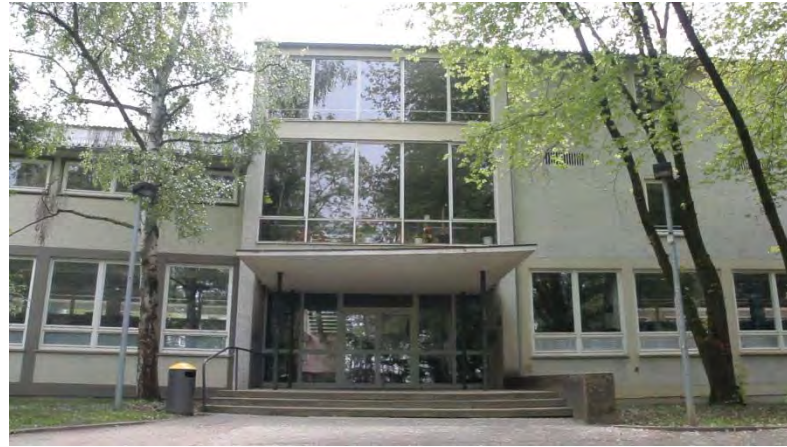
Nordfassade North facade
