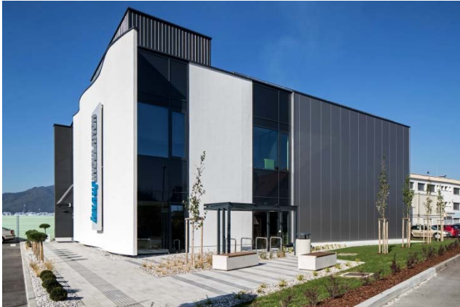
Knauf Insulation Experience Center Škofja Loka
