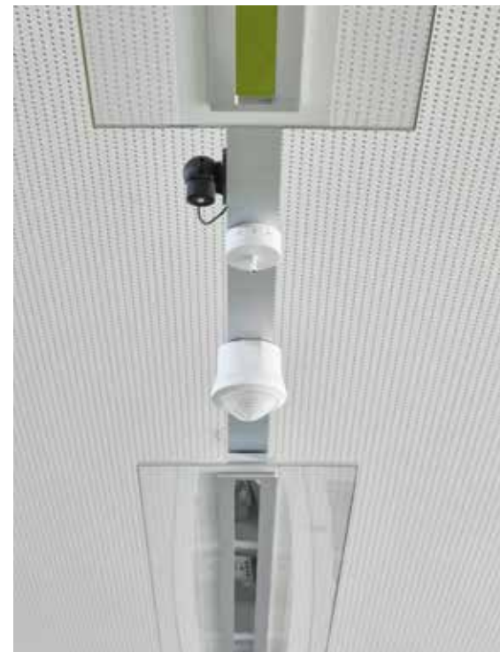
Black sensor: photometer head to measure illuminance
