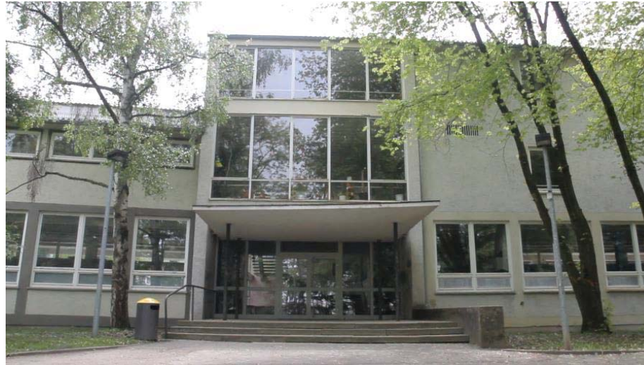
Nordfassade North facade
