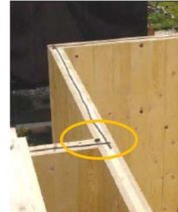
Connection of longitudinal wall to transverse wall:
